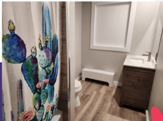
Bathroom Renovation - After
