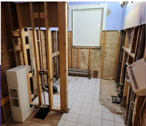
Bathroom Renovation - During
